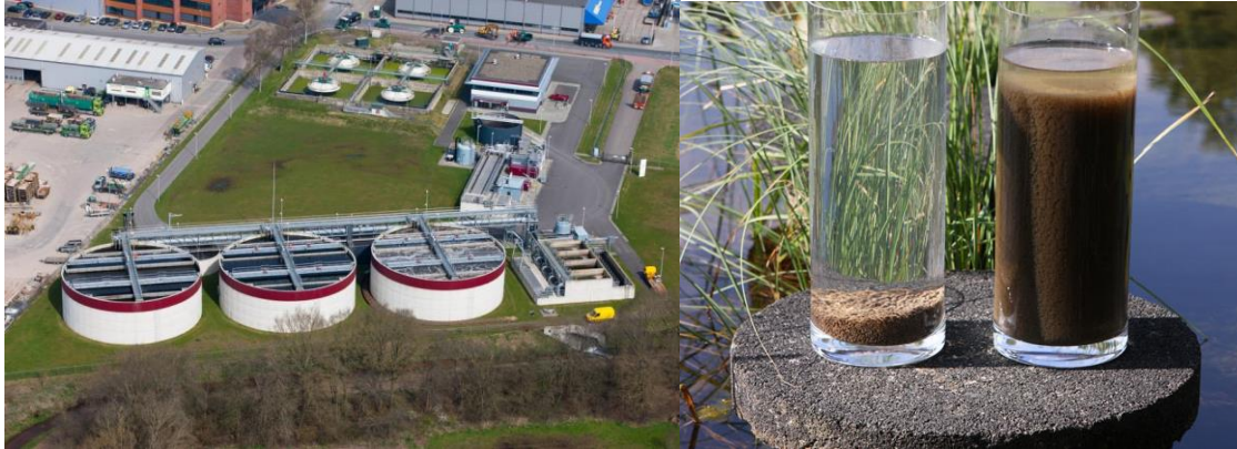
Figur 25 Nereda® fuldskala installation, Epe WWTP, Holland
