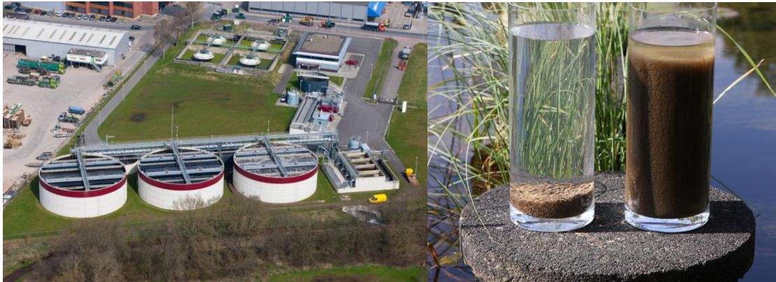
Figur 25 Nereda® fuldskala installation, Epe WWTP, Holland
